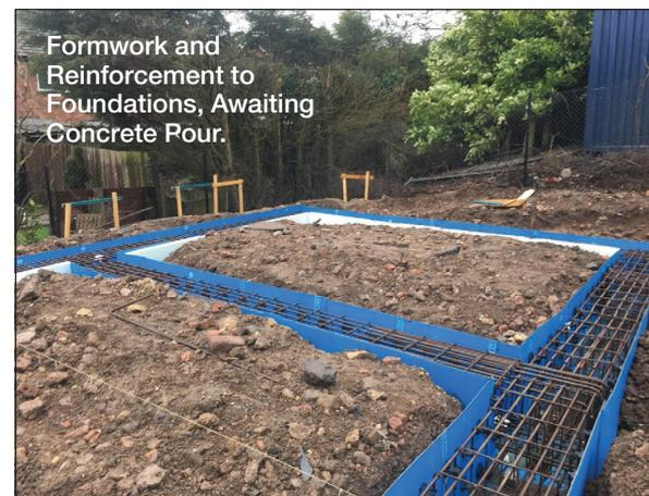
Formwork and Reinforcement to Foundations, Awaiting Concrete Pour.
